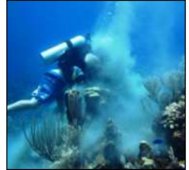
Adding cement to stabilize grounding
