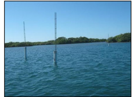
Illegally constructed pylons in Dixon Cove
